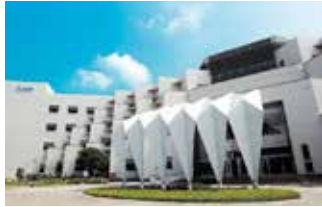
Tainan Plant (Diamond-rated Green Building)
